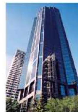
Centerra Tower, Calgary, Canada LUNDHS Royal Blue, facade.
