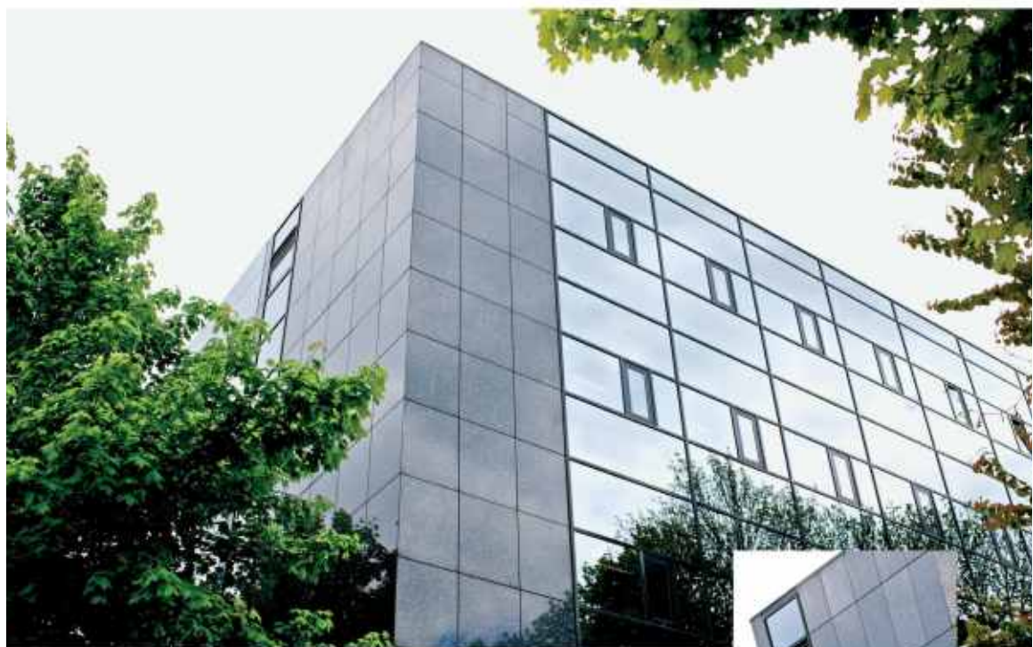
Office building, Norway. Stone: LUNDHS Blue.
