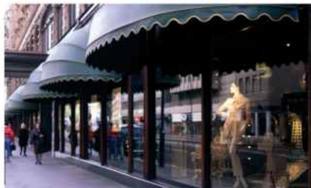
Hamods, London, UK LUNDHS Emerald, facade & ground floor shop front.
