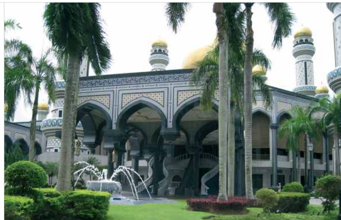
Jame'Alr Hassanah Mosque LUNDHS Blue on columns, stairs and arches.
